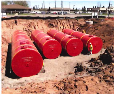
Underground Storage Tank Installation
