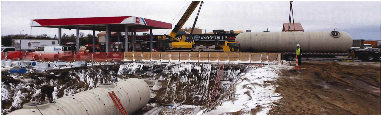
Underground Storage Tank Installation
